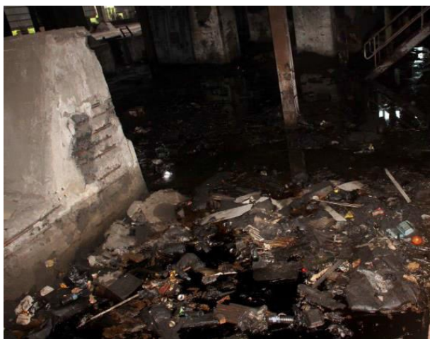
Fig 4 A: Pool of possible PCB oil with contaminated solid debris
